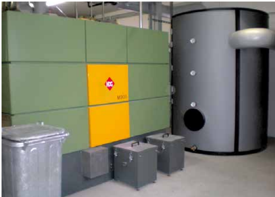
The M300-400 is often equipped with an accumulator in practice. The speed-regulated accumulator heating pump provides for a particularly effective output and delivers the appropriate flow volume in the complete output range.
